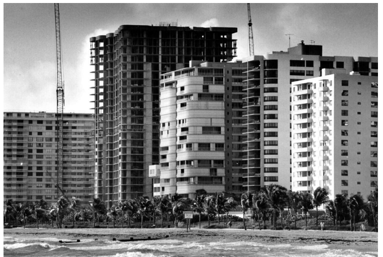
Bal Harbour Tower under construction among other condos in Bal Harbour. Randy Bazemore Miami Herald File
