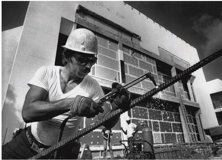
Michael Quirello cuts steel with a blow torch for the expansion of Saks Fifth Avenue in Bal Harbour. Randy Bazemore Miami Herald File
