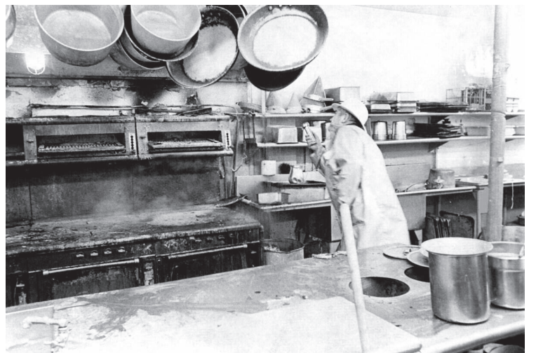
A firefighter inspects damage after a blaze at the Singapore hotel in Bal Harbour. Battle Vaughan Miami Herald File
